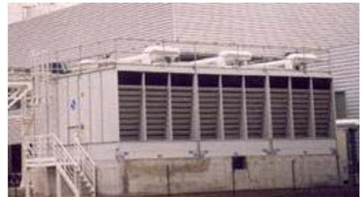
Typical induced draft, cross-flow cooling tower.
